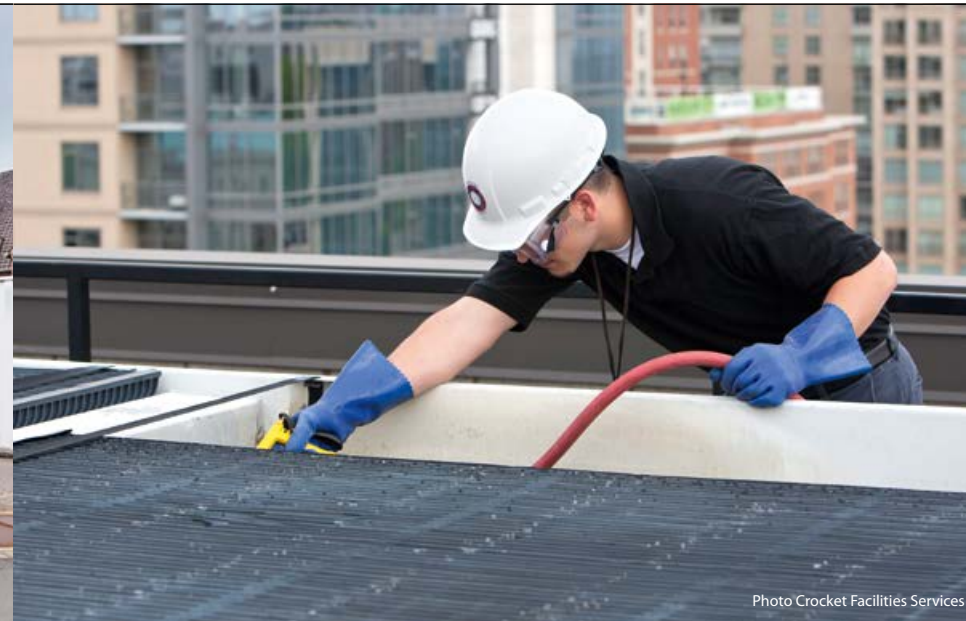
Photo Crocket Facilities Services
